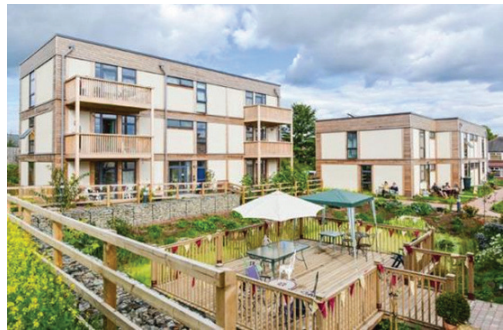
Fig. 5. LILAC (West Leeds, UK) – ecological co-housing with twenty flats consisting of detached blocks of flats and a community house
