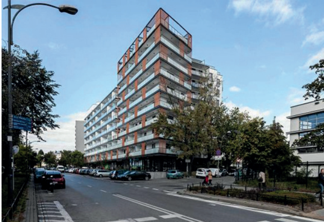
Fig. 3. The building housing the Model Senior Residence (WMS) fully adapted to the needs of people with disabilities
